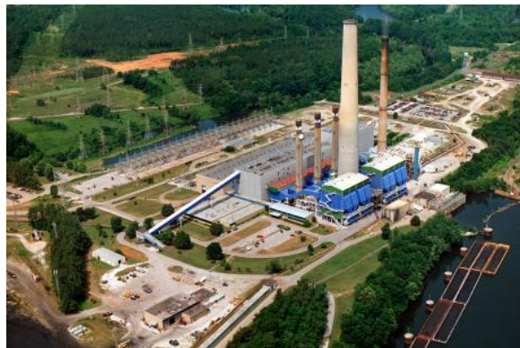
TVA Colbert Power Plant Huntsville, AL - DEC 1998
